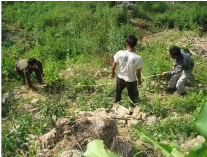
Measurement for the protection and stabilization wall
