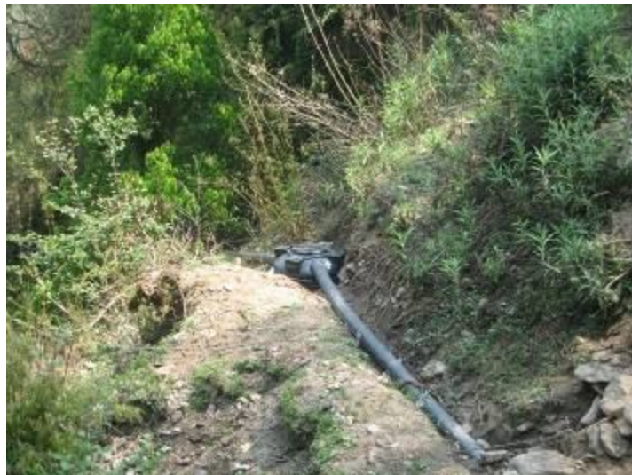
Water tank and pipes
