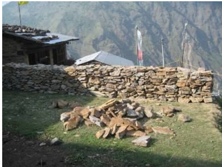
Stones for the protection wall
